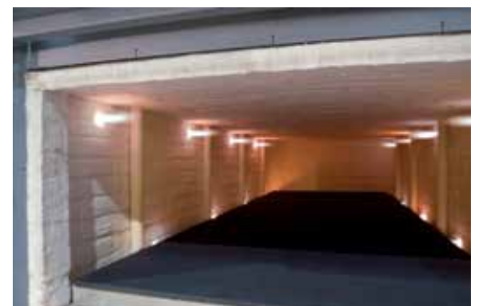
Furnace chamber with eight high-speed burners
